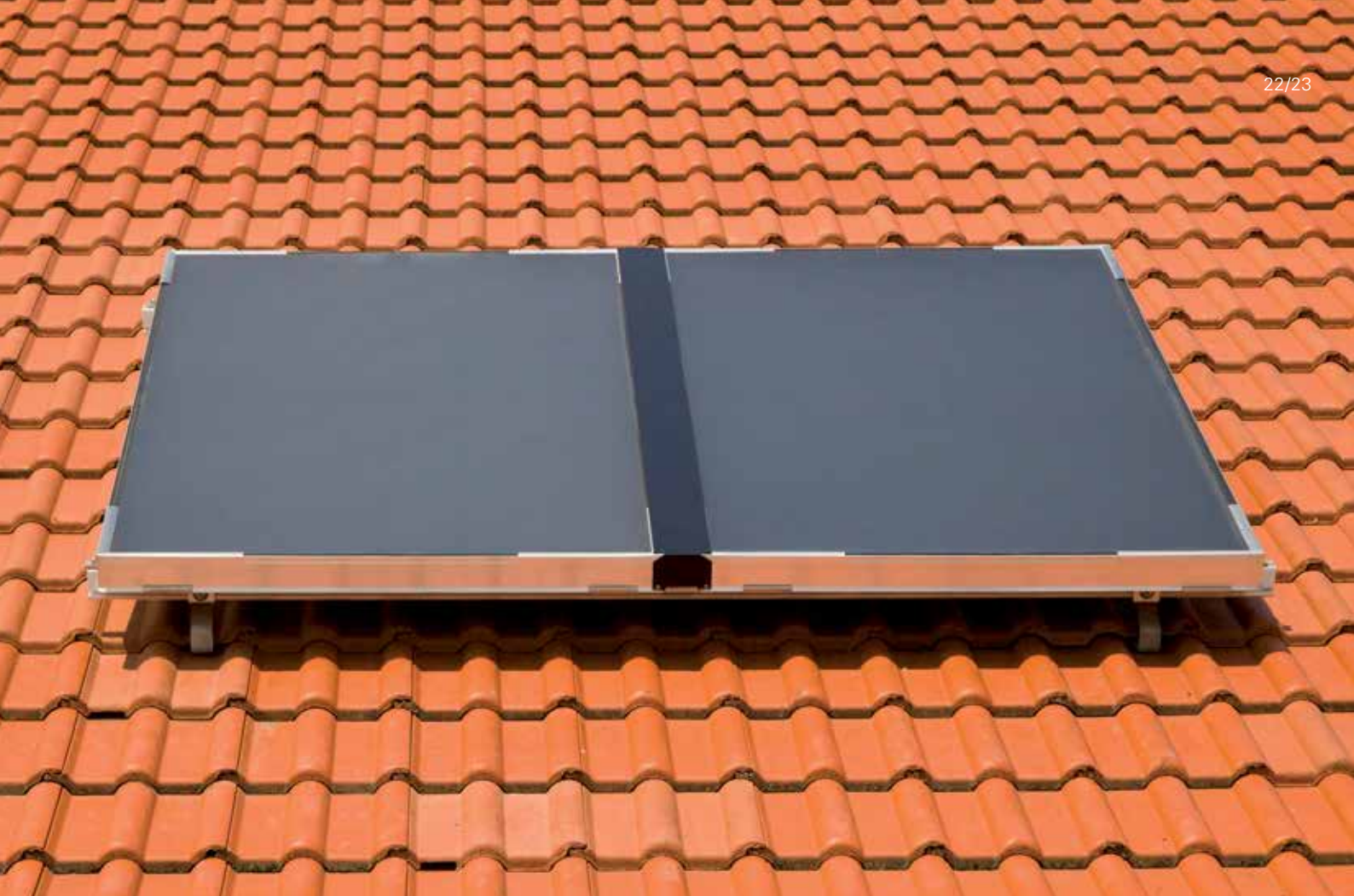
Vitosol 100-FM twin panel pack fully installed
