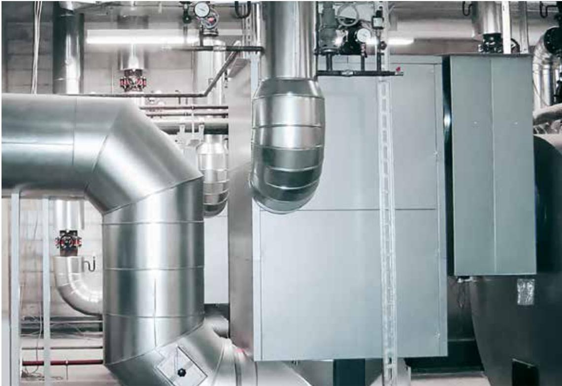
Downstream Vitotrans 300 heat exchanger fitted to a Vitomax boiler
